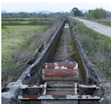
A sluice gate on one of the main channels supplying water for flood irrigation, near Karditsomágoula
